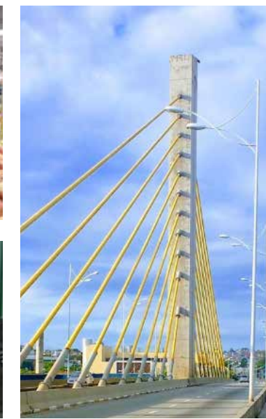
Ponte Akira Hashimoto
